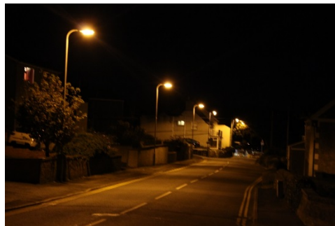
Figure 1-3 Bridge Street, Cemaes. High pressure sodium street lights (left, October 2016) LED lights installed with tilt (right, January 2018)
